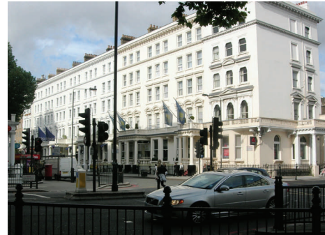
Above: Cromwell and Gloucester Roads intersection
